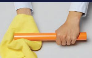
3 Wipe with clean cloth to remove any dirt, grease, or moisture
