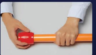
2 Deburr and Bevel the pipe to ensure a smooth surface
