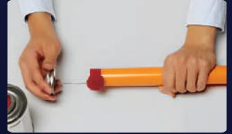
5 Apply CPVC Solvent Cement using a dauber to the pipe 2-3 times
