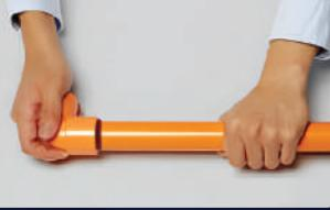
7 Insert pipe to fitting while turning 1/4 and hold for 30 seconds
